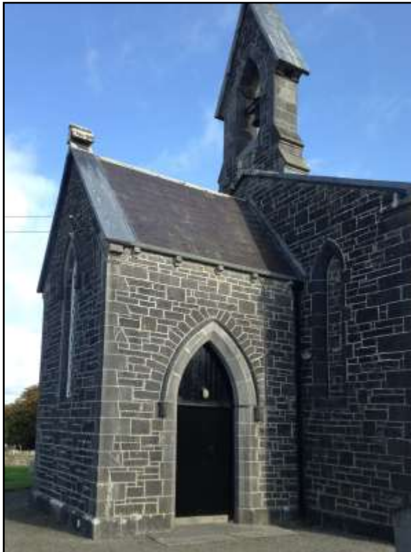
The freshly repainted Annatrim Church door
